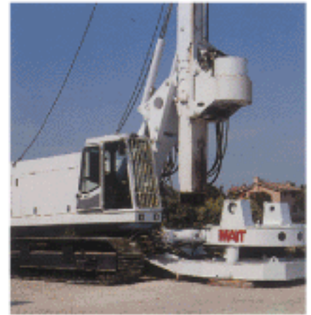
Large bore piles with casing oscillator
