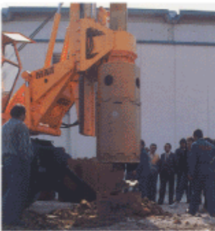
← Drilling with casing tubes
